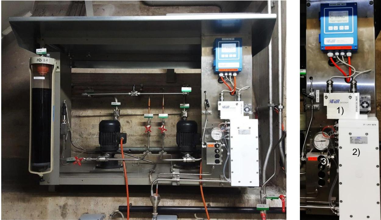
Figure 7: Installed conductivity instruments in the condenser hotwell in Beznau NPP
