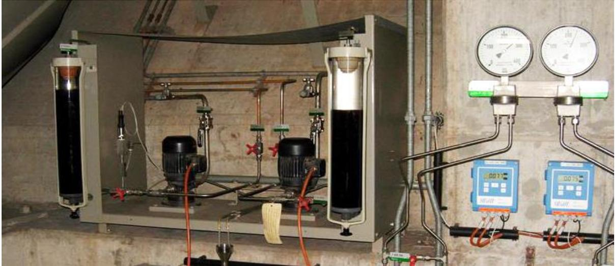
Figure 5: Hotwell monitoring station in Beznau NPP with conventional cationic exchanger resins, to the left turbine side of the hotwell and to the right the generator side.
